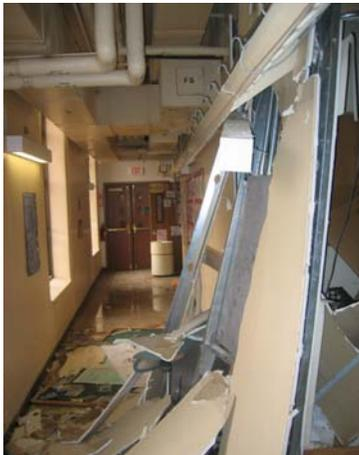
Figure 2 - Hallway Outside Laboratory Showing Explosion Damage
