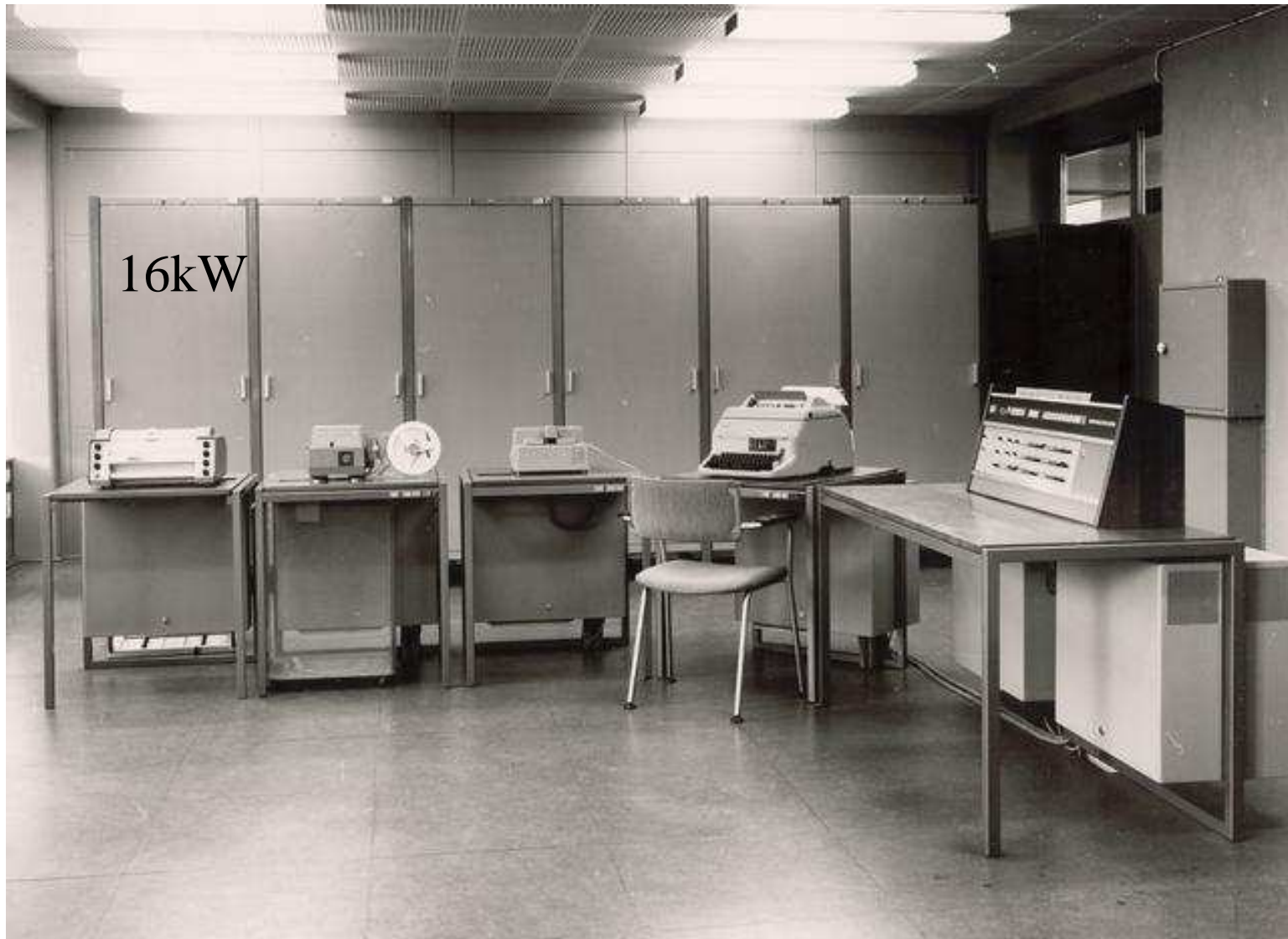
~1966, Electrologica X8 ALGOL60 'Mainframe' (<1MHz)
